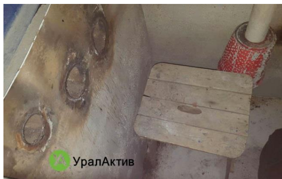
Vessel before lining by PP
